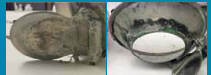
Before: Inorganic buildup typically found on lavatory flapper and components
